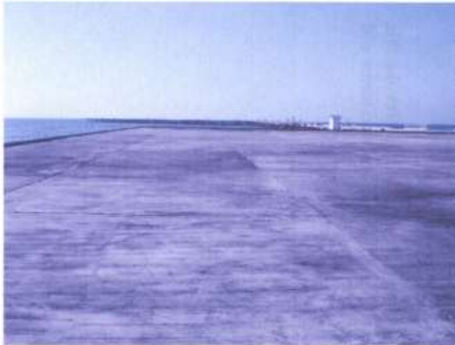
Concrete Back-up Area Area = 3,840 sq. m. (Port of Curimao, Ilocos Norte)
