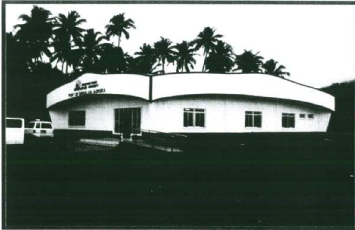
PASSENGER TERMINAL BUILDING (PTB) - (262.8 sq. m.) RESERVED FOR FERRY OPERATOR Port of Dingalan, Brgy. Aplaya, Dingalan, Aurora
